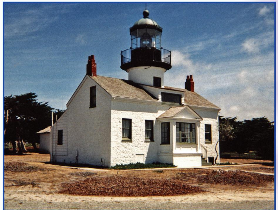
lens has been guiding ships since 1855. A whale-oil lantern was the first light source, and then lard oil and kerosene were used. In 1915, electric light was installed. Now a 1000-watt bulb is amplified by the lenses and prisms, producing a beam that can be seen 15 miles out to sea.
